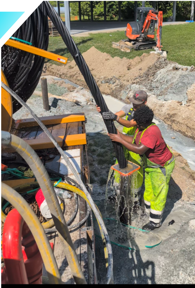
Installation of 17 Twister Geothermal Loops
